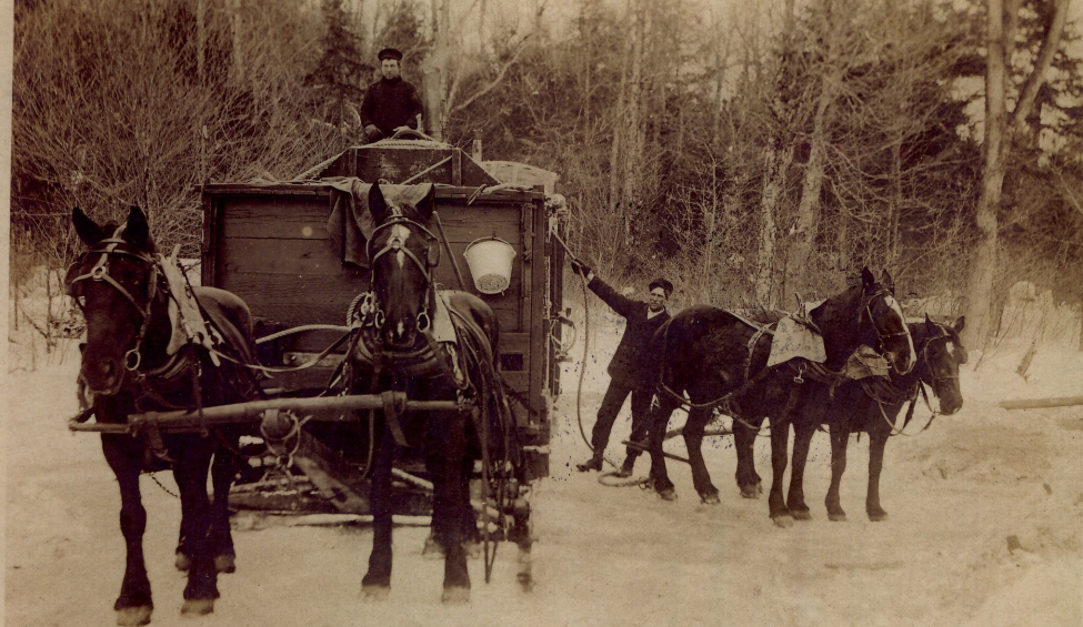
FILLING THE TANK.
